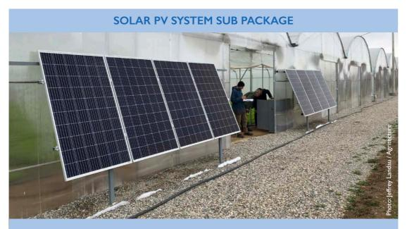
The Solar PV sub package is designed to generate electricity to operate any mechanical devices associated with agribusiness operations. Assuming a 1,000 m² greenhouse, a 10 kWp system is recommended. The estimated cost, including installation, for a 10 kWp system is approximately epsilon7,500 and the payback period is roughly 6-7 years, assuming that the operator is connected to the grid and able to take advantage of net metering.
